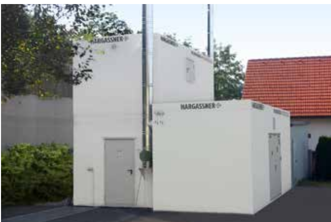
Triple-floor heating module in a catering operation.
