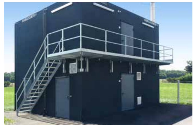
Quadruple wood chip heating module for an industrial building.
