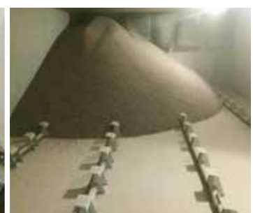
Fuel storage for 120-t pellets
