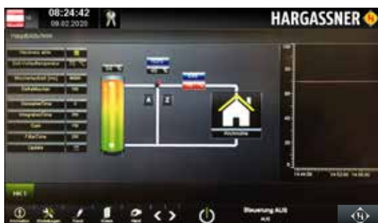
Control of external buildings
