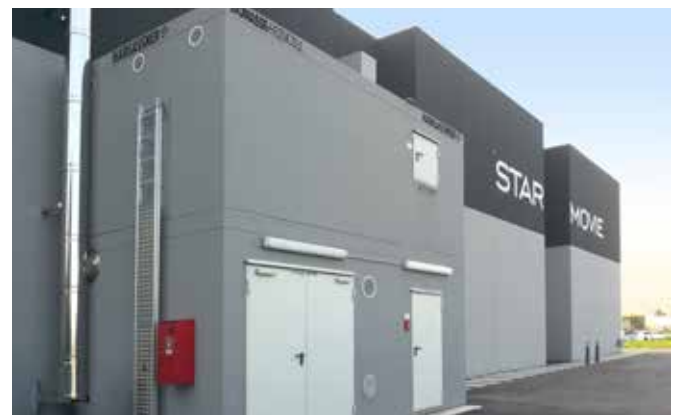
Double-floor wood chip heating module next to a public building.
